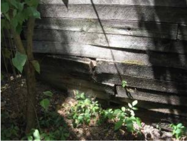
Decayed retaining wall at South side
