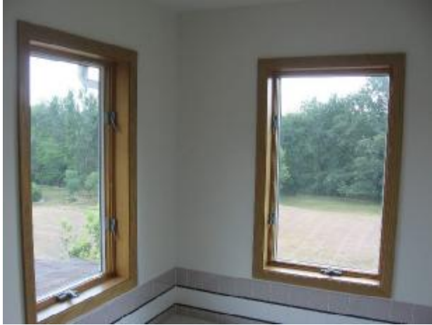
Replace with tempered glass
