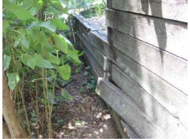
Decayed retaining wall
